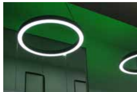
CIRCUS + | Ring-shaped suspended pendants with a direct-indirect light distribution providing 3000K direct and RGB indirect lighting. Seen here in 1200mm, 1500mm and 2500mm diameters.
